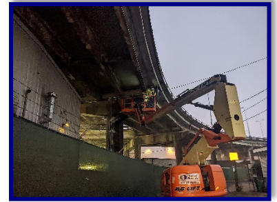
Causeway Blvd. Overpass at Airline Drive
