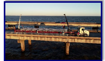
Causeway Bridge Rail Improvements
